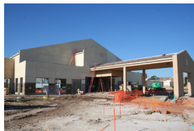
Community Living Center exterior during construction
