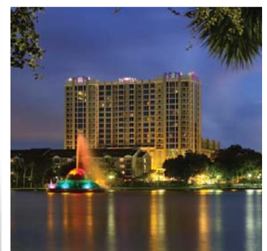
Paramount on Lake Eola. 16-story tower with 313 condos, parking, retail and grocery store. Chilled water systems. Installed mechanical value = $4.5 million.
