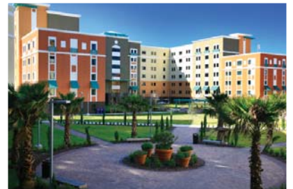
UCF Student Housing at Knight's Plaza. 2,000 beds within 4 buildings, 3 parking garages, retail space. 2 miles underground chilled water lines. Mechanical value = $8 million.
