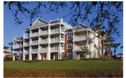
Villages at Reunion Square. 36 buildings with 504 condos, 4 maintenance buildings, parking areas. 508 DX split systems. Mechanical value = $8 million.
