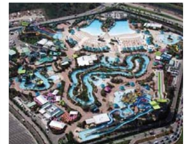
Aquatica at Sea World Orlando. Provided design-assist HVAC services for 124,500 square feet with approximately 500 tons of cooling. Installed mechanical value = $2 million.
