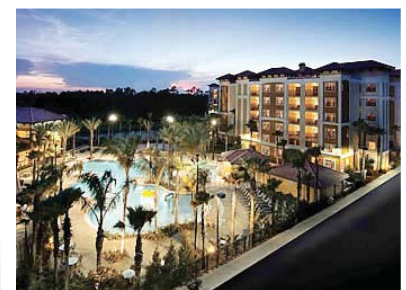
Floridays Resort. Completed HVAC scope for six, five-story hotel buildings, welcome center and maintenance building. Approximately 450 units of various sizes. Installed mechanical value = $1.8 million.
