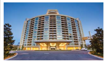
Bay Lake Tower at Disney's Contemporary Resort, Kissimmee, FL. 15-story, 525,000 sq ft high-rise 428-guestroom timeshare resort. Installed mechanical value = $8 million.
