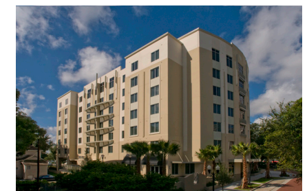
Orlando Lutheran Tower
